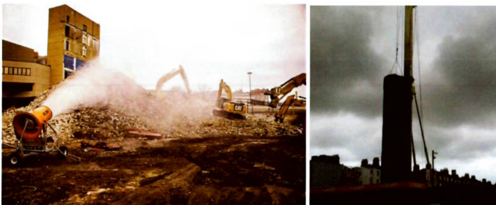
Figure 40 – Typical Dust Mitigation Measures
