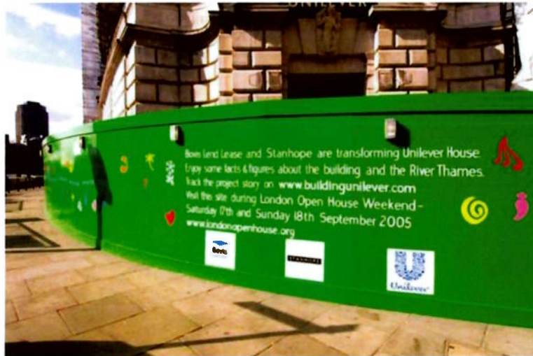
Figure 5 Typical Pavement Hoarding with Street Lighting
