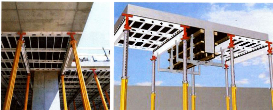
Figure 14 - Typical RC Formwork (Skydeck)
