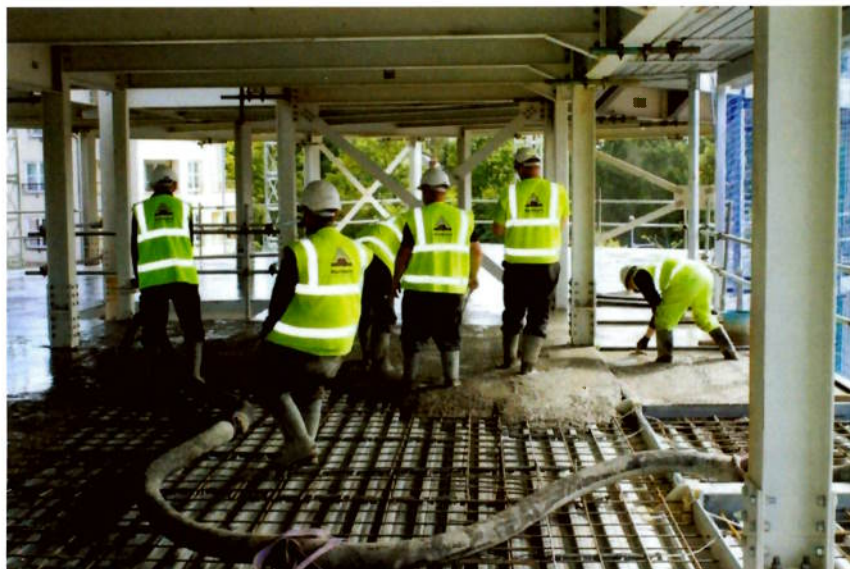
Figure 17 – Typical Concrete Pour on Metal Decking
