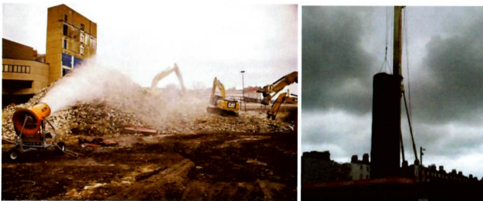
Figure 26 – Typical Dust Mitigation Measures
