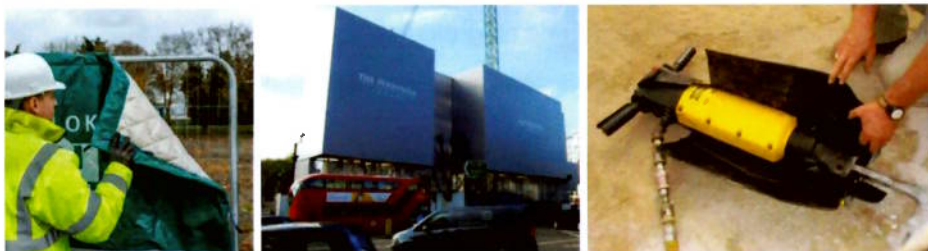
Figure 26 – Typical Noise Mitigation Measures
