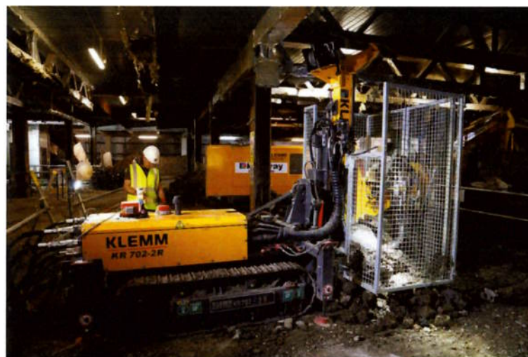
Figure 12 – Typical Mini-Piling Operation
