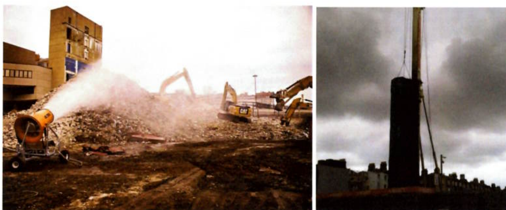
Figure 27 – Typical Dust Mitigation Measures
