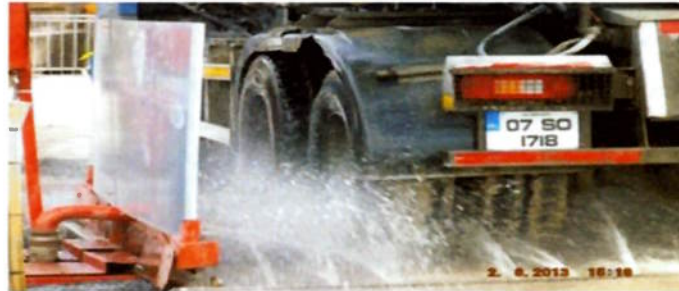
Figure 9 – Typical Wheel Washing Facility
