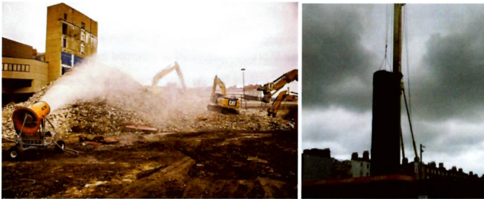
Figure 16 – Typical Dust Mitigation Measures
