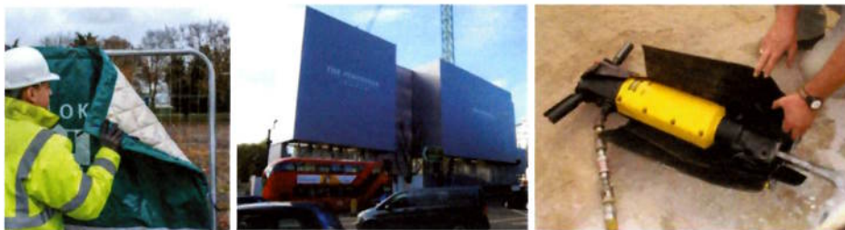
Figure 25 – Typical Noise Mitigation Measures
