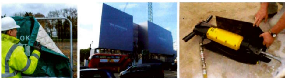
Figure 15 – Typical Noise Mitigation Measures
