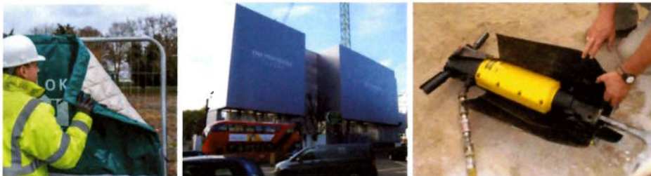
Figure 39 – Typical Noise Mitigation Measures
