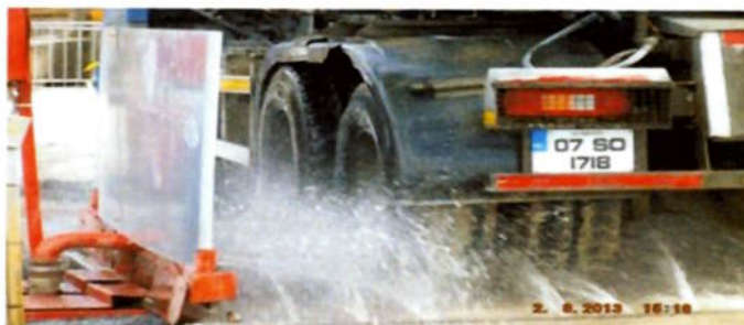
Figure 8 - Typical Wheel Washing Facility
