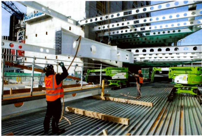
Figure 16 – Typical Steel Frame Erection
