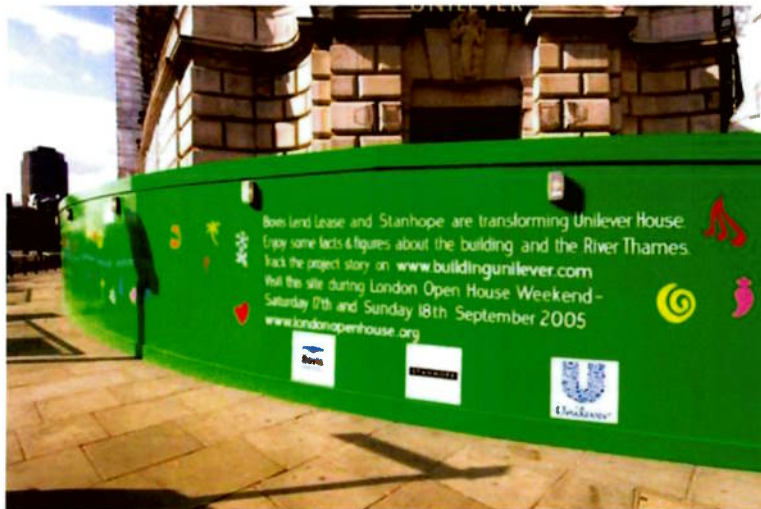
Figure 5 – Typical pavement hoarding with street lighting
